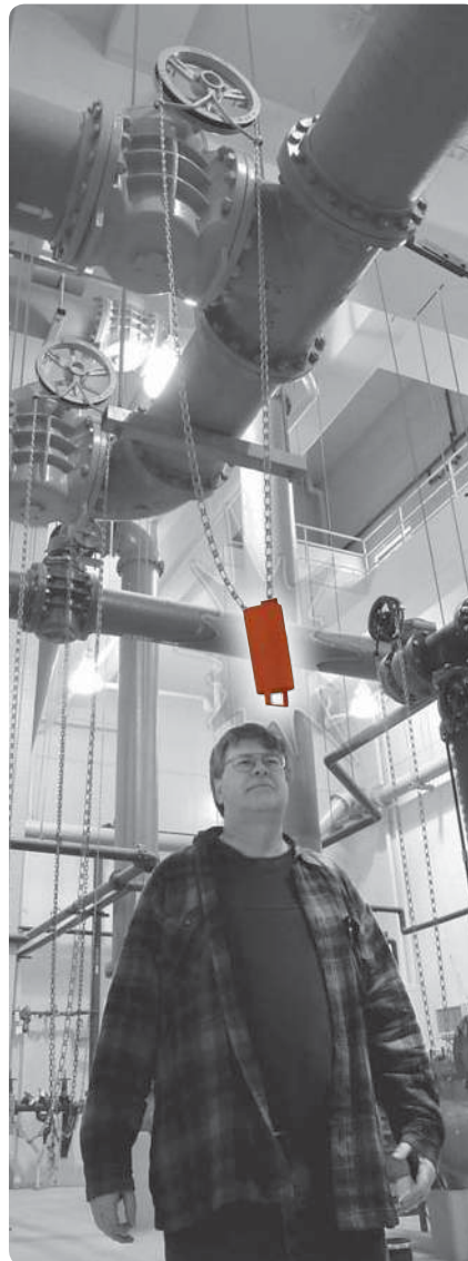
CHAIN-UP DEVICE stores the chain above pathway.
